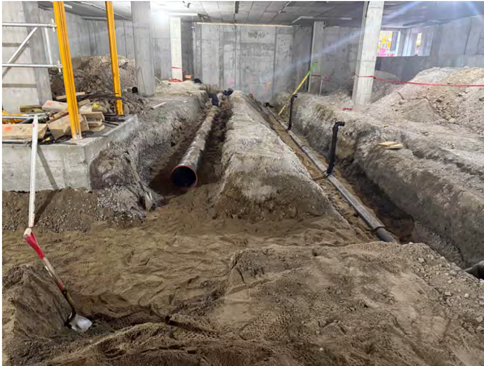
Underground plumbing, Building A garage level, 11/10/25
